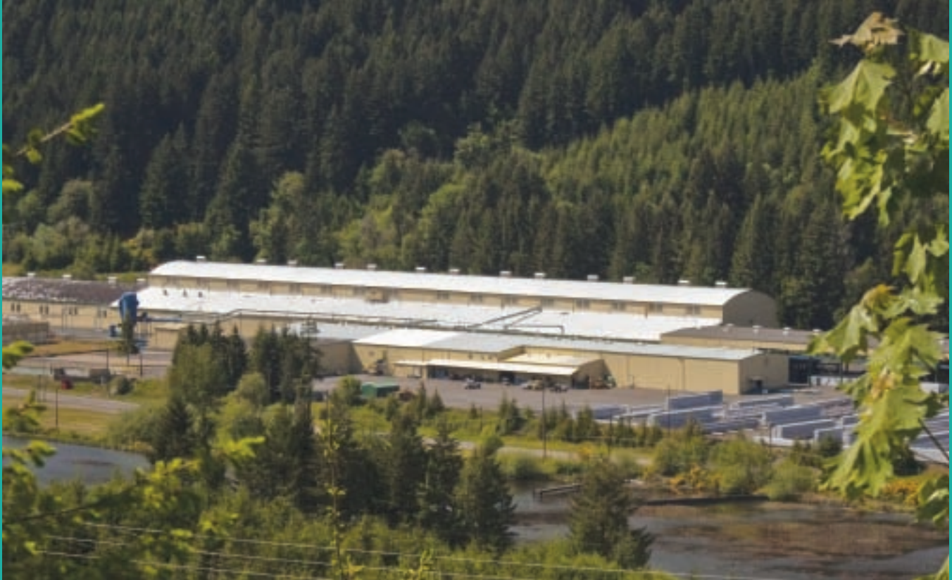
Rosboro's Glulam plant in Vaughn, Oregon
