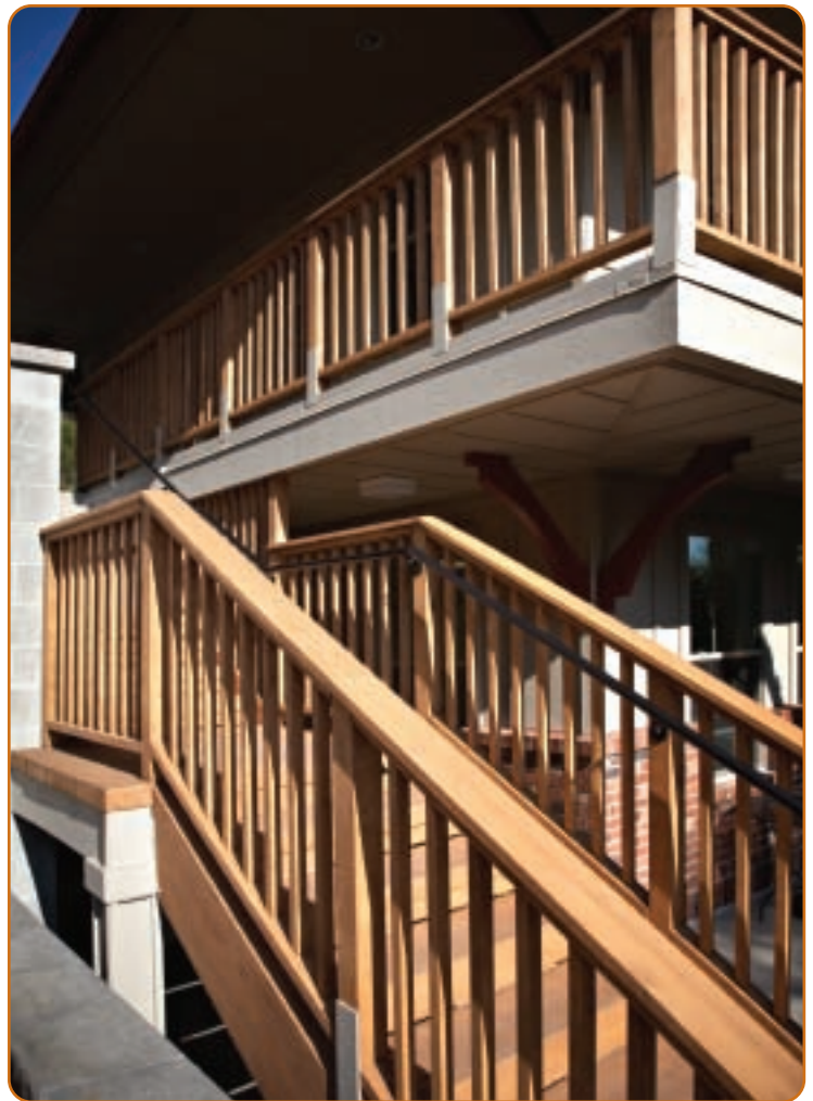
Yellow Cedar posts and rails.
