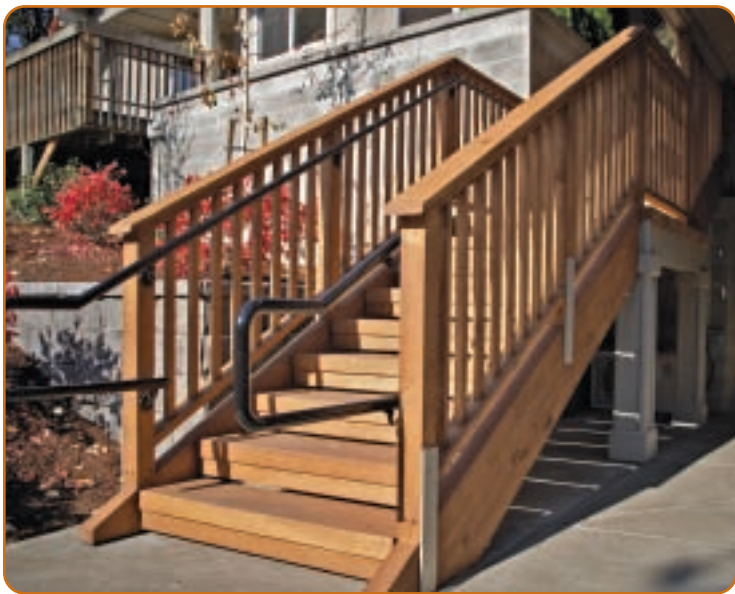
Alaska Yellow Cedar glulam was used for both the steps and the stringers.
